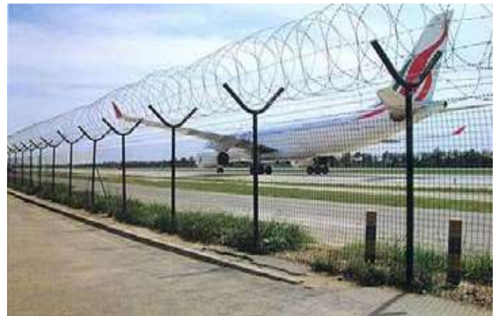
Figure 4 Well-maintained fence, no gap at the bottom
