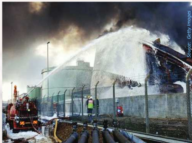
The petroleum industry has long relied on AFFF to snuff out fires at facilities worldwide, on both land and sea. Here, firefighters in the United Kingdom spray foam onto oil storage tanks during a fire at a depot on the outskirts of London.
